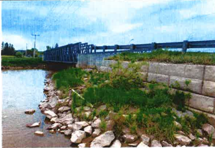
Photo Description Concrete block retaining wall at north approach.
