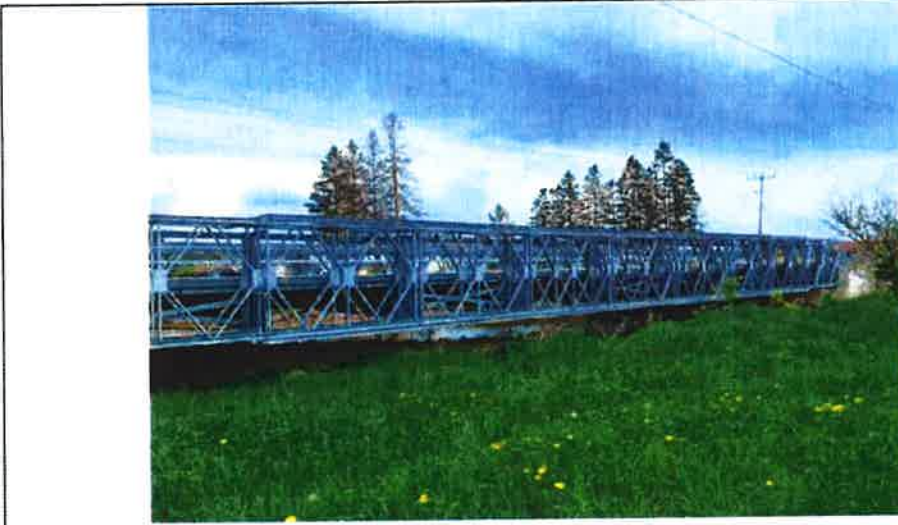
Photo Description Downstream façade.
