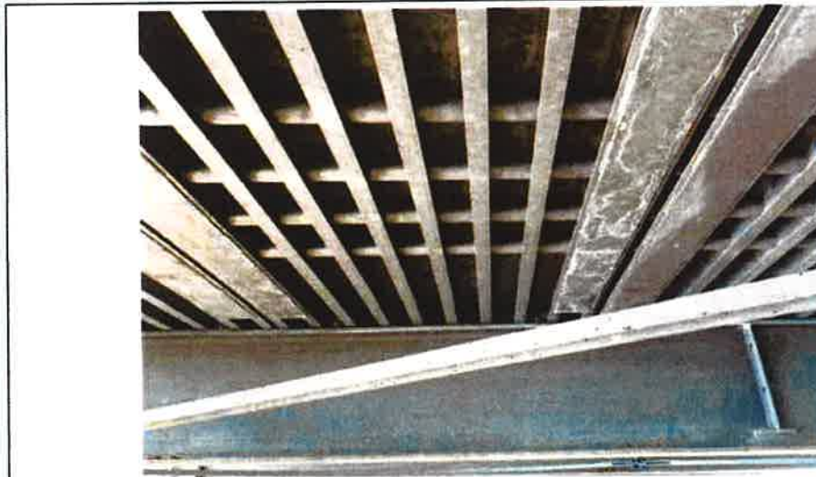
Photo Description Typical condition at underside of deck.
